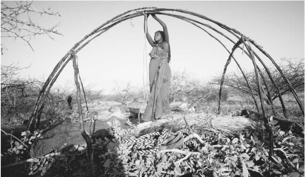
A Somali nomad woman ties roof supports together to reconstruct a portable hut after moving to a new location. The aqal is easy to break down and reassemble.
